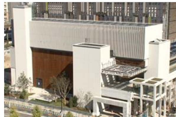
Decentralized Energy System in Tamachi
