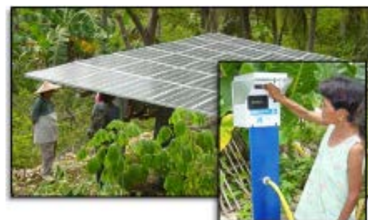
Figure 14 Prepaid underwater pumping system (Source: Aquameter)
