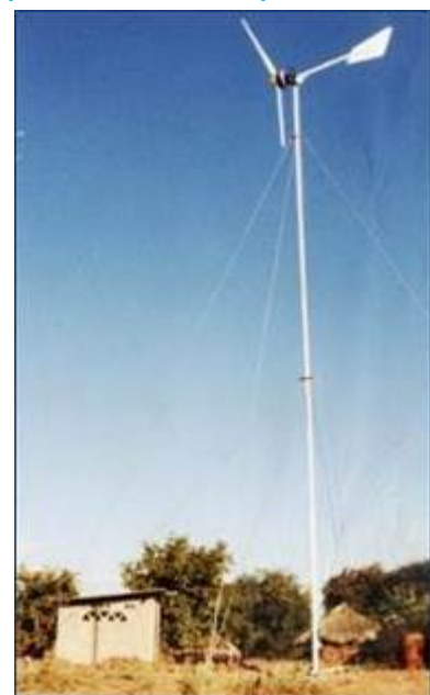
Figure 30 Small Wind Power plant in Zimbabwe (Source: AfriWEA)
