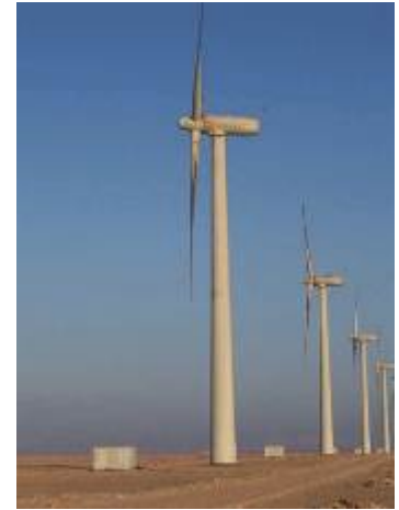
Figure 29 Zafarana 430MW wind farm in Egypt (source: NREA, Egypt Govt.)
