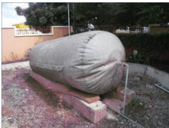
Figure 39 A Biogas plant at African Regent Hotel in Accra (19th September 2010, photo credit: Author)
